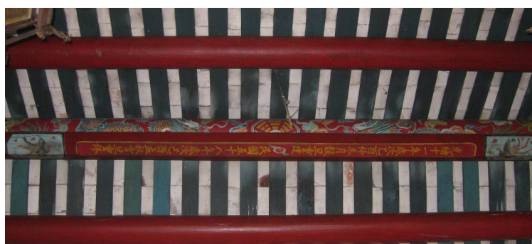
Picture 3. The main purlin at Teochius huiguan in Hoian, dated in 1885 and 1969
